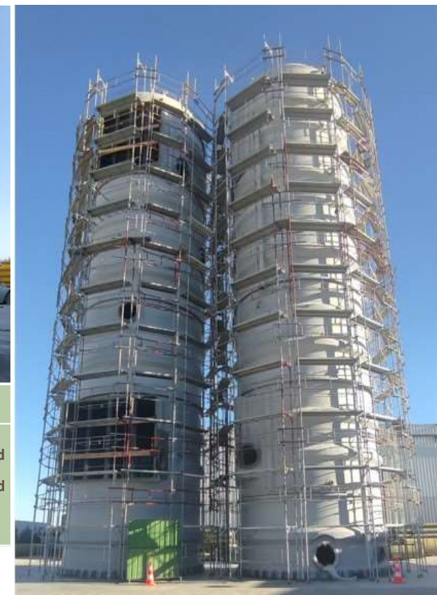
Trial assembly of condenser DN6500 (2 lines )
