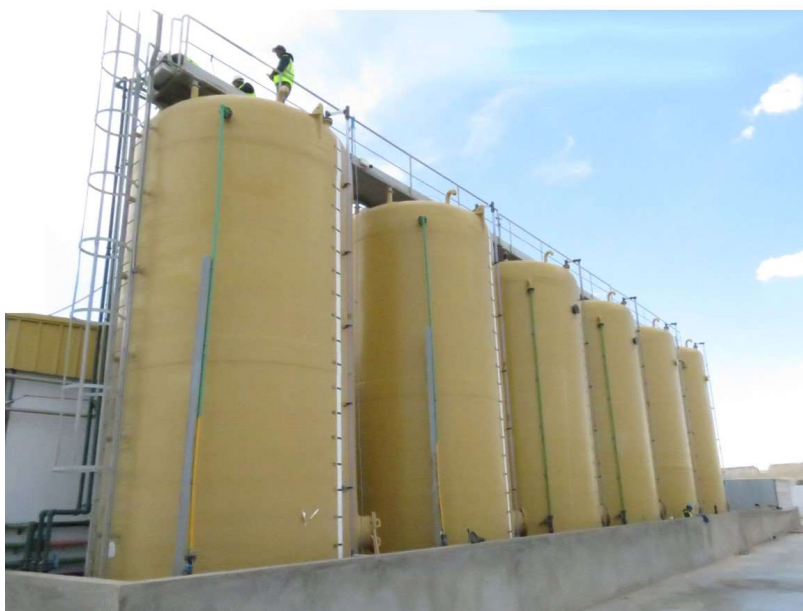
SODIUM HYPOCHLORITE STORAGE TANKS
