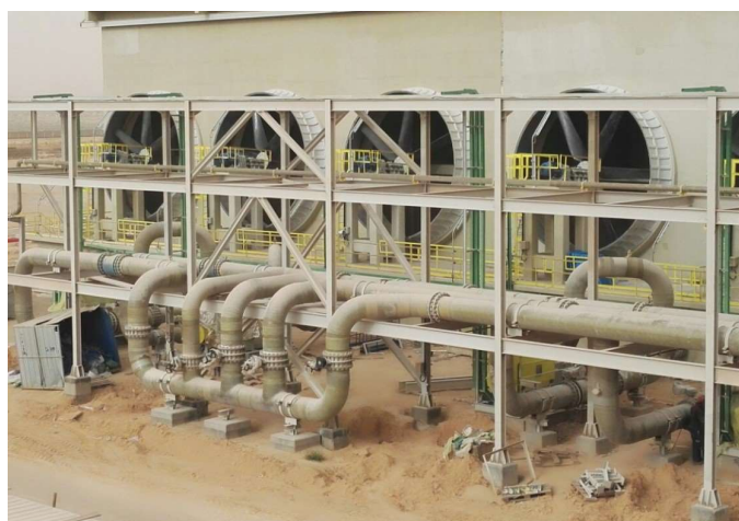
GRP PIPE INSTALLATION
